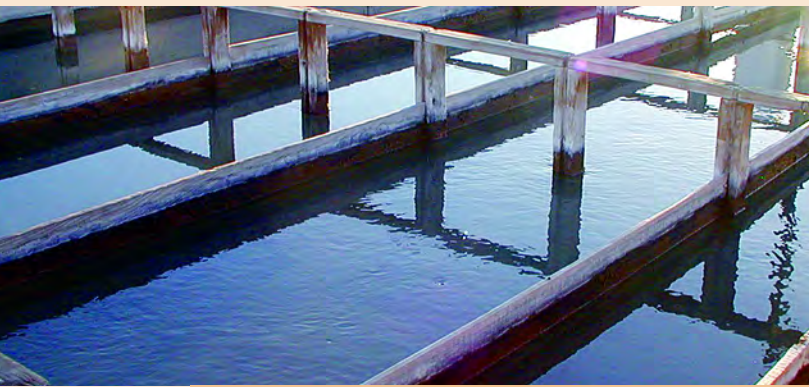
Wastewater treatment plant in Seeley, California
